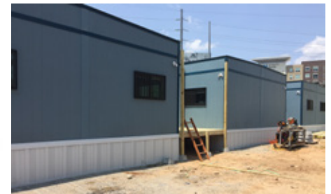
Installation of decks and ramps underway
